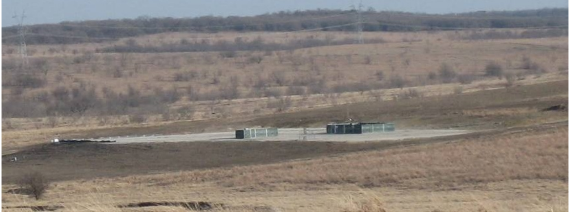
Figure E.2. Gas well site on modified hillside
